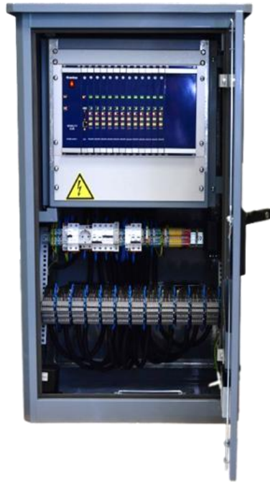
Figure 14: ACISA's next-generation traffic light controller integrates edge computing capabilities to support the deployment of containerized applications (i.e., V2X services, Video analytics, etc).
